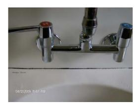
The sink in the dirty utility had a broken seal, this should be replaced as it cannot be cleaned effectively and this can cause a potential risk of contamination.
