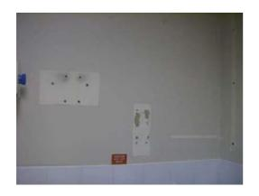
Within the dirty utility and sterile store room items had been removed from the walls leaving visible holes, these should be filled so that the areas can be cleaned appropriately.
