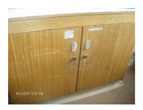
The cupboards in the treatment room were wooden and should be replaced. Wood cannot be cleaned effectively and hence there is a potential risk of contamination.
