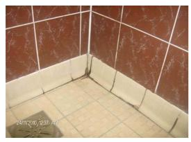
The tiles in the shower room were in a poor state of repair, making it difficult for them to be cleaned appropriately.
