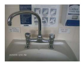
The hand washing sinks in the treatment rooms were not acceptable as the taps are incorrect and do not conform to Health Technical Memorandum (HTM)
