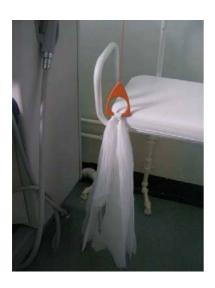
In the bathroom an apron had been attached to the emergency call as the length of the call bell was too short. This is unacceptable due to the risk of contamination. This should be removed and a suitable length string fitted so that the emergency call bell is long enough.
