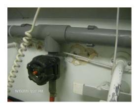
A number of pipes have been moved on the ward and as a result there are holes and bare plaster, this is unacceptable: all holes of bare plaster should be recovered.
