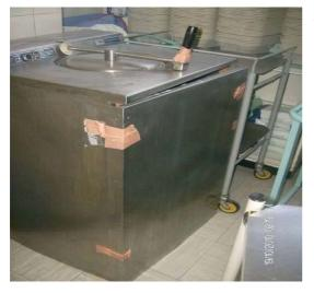
• The macerator in the dirty utility was found to be in a poor state of repair and being held together with tape. This is unacceptable as there is the potential for contamination as the macerator cannot be cleaned effectively.
